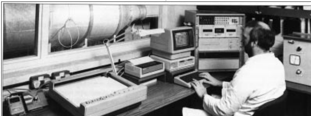
Computer-automated fan test room.
